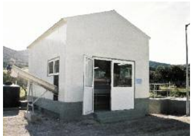
The biological waste treatment plant at Aghia Styliani
